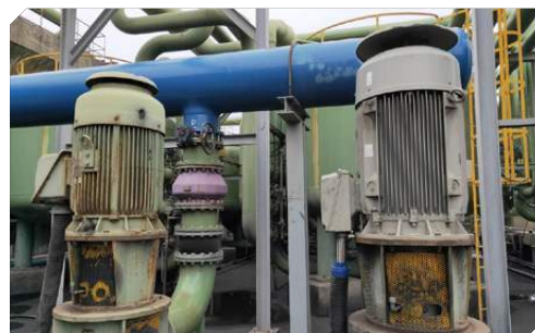
A new inverter motor was installed in Taoyuan Works (On the left is the general motor and on the right is the inverter moto.)
