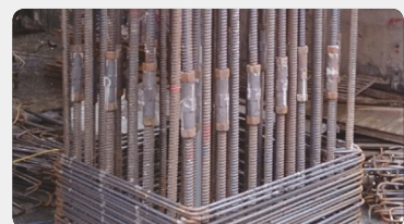
Assembled Screwed Re-Bar couplers
